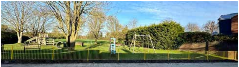
Chequer Street – Hedges removed, and new Fencing being installed.
